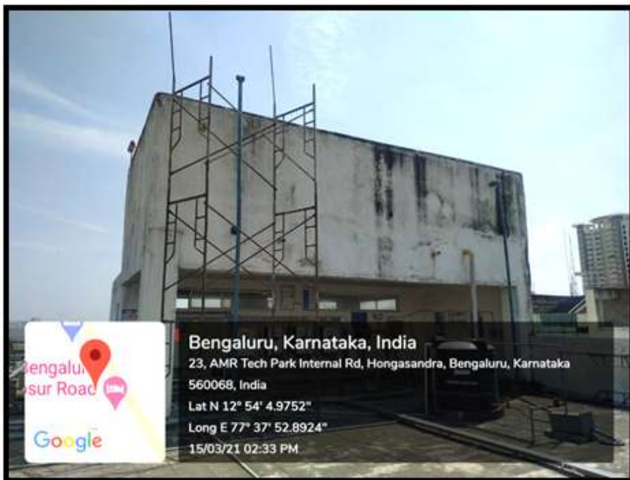
Overhead tank in the Old building
