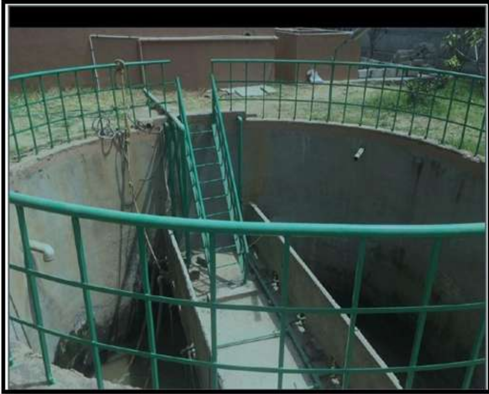
Recycling of waste water process
